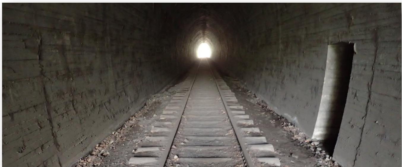
*Retention of the unique hog's back timber railway sleepers within the tunnels is one of the key factors to be considered when developing the rail trail.*
