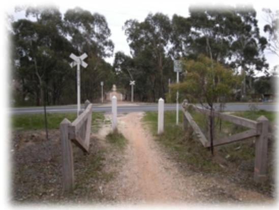
*Various techniques are available to make road crossings safe for trail users, including this simple technique used on the O'Keeffe Rail Trail (in Victoria). On other rail trails, road crossings have been made safer by the installation of underpasses, bridges and traffic lights.*
