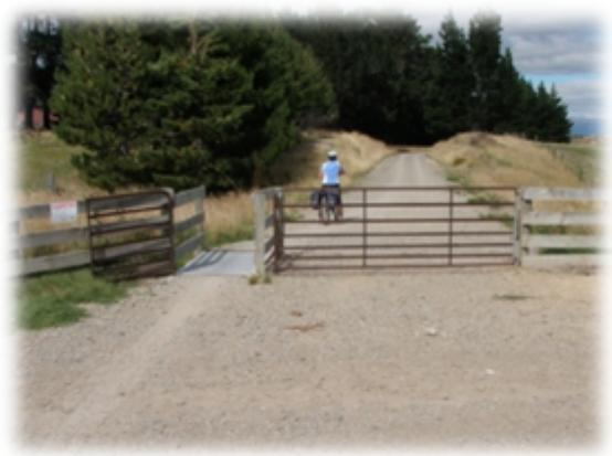
*Grids are commonly used on rail trails at fence lines and property boundaries to prevent stock from escaping, but still allowing the passage of cyclists and walkers. This example is from the Otago Central Rail Trail in New Zealand. Similar examples can be found on the Brisbane Valley Rail Trail and the High Country Rail Trail in Northern Victoria.*
