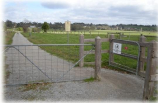
*The gating system at road crossings used on the Lilydale Warburton Rail Trail in Victoria makes it difficult for unauthorised users (such as motor bikes and 4WD vehicles) to gain access to the rail trail.*
